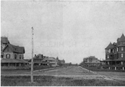
From the collection of John Russell (1895 photograph of Mercer Avenue)
